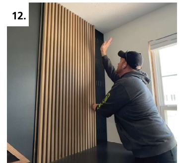
12. Snap slats into place on finished project
