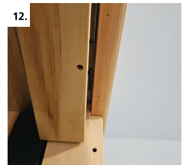
Repeat all steps above (except for back-beveling) to install header jamb Use cover caps if desired
