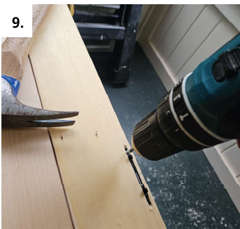
Screw each connector half into place (both screws at same time to keep alignment centered)
