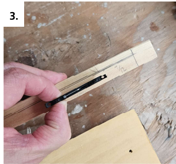
Determine slot position in jamb and casing
