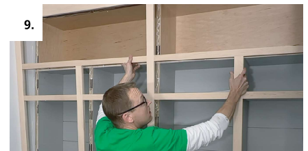
9. Install face frame
