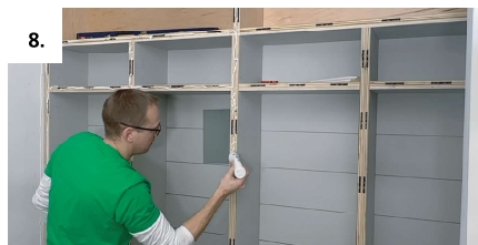
8. Apply glue (when using Tenso)
