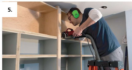
5. Cut corresponding slots on cabinet boxes
